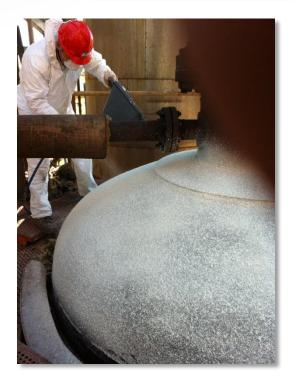
Application of HOT PIPE COATING = 9.9mm thick with a hopper gun
